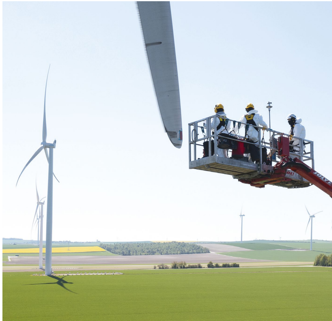
Wind turbine maintenance © 2022 Petzl Distribution - Vuedici.org - GR Wind - Vestas - Joly - EDF Renewables - Les Coteaux wind farm
