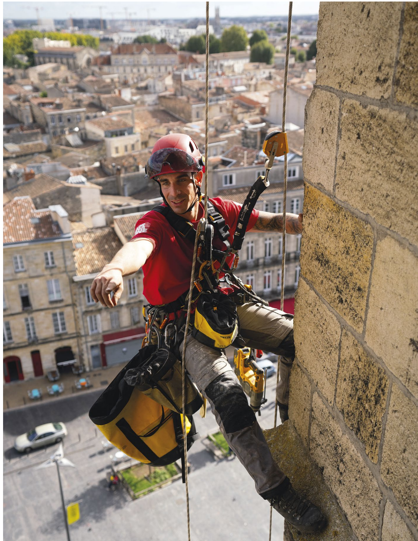
Installing monitors on the spire of the St Michel Church, Bordeaux, France © 2021 Petzl Distribution - Vuedici.org - Adrénaïne - Bordeaux City Hall
