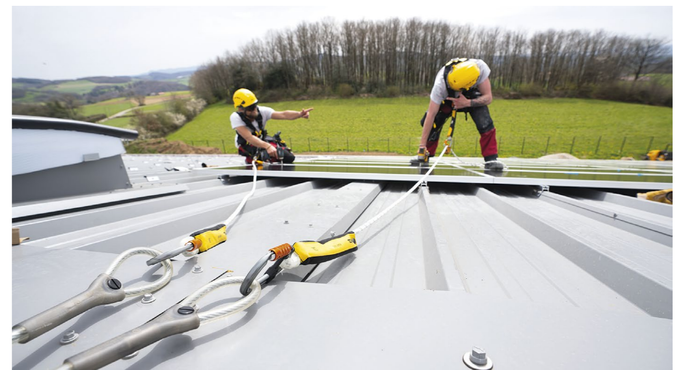
Solar panel installation, France © 2022 Petzl Distribution - Vuedici.org - Laurent Moretton
